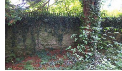
Item: Stone Boundary Wall Comments: Stone and plaster to 2.5m ht.; compromised at several locations Category: 5
