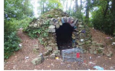
Item: Ice House Comments: Style and setting, intact but used as a rubbish dump and graffitied Category: 5
