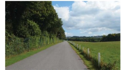
Item: Tarmac Entry Avenue Comments: Alignment and scale Category: 3
